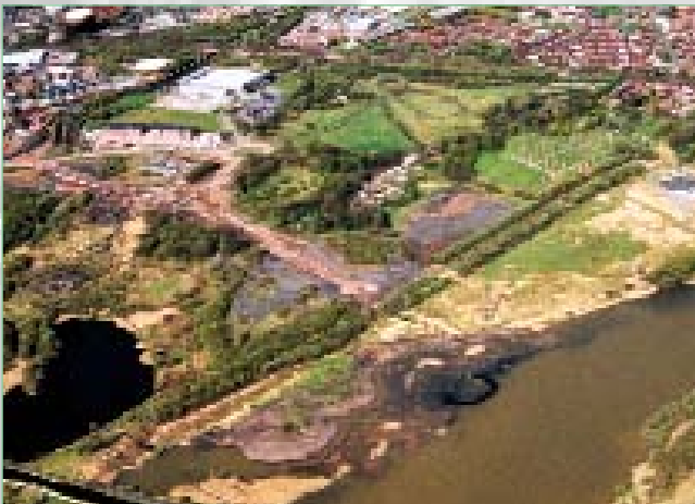
Phase 1 infrastructure works at Westwood Park
